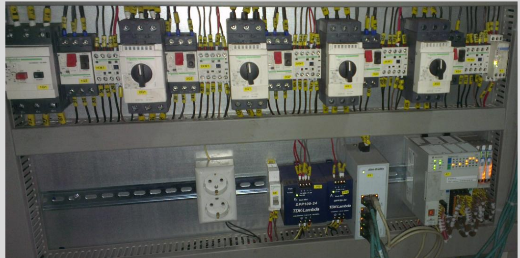
Electrical panels for crane with relay – contactors control and with frequency invertors in network communication with PLC.
