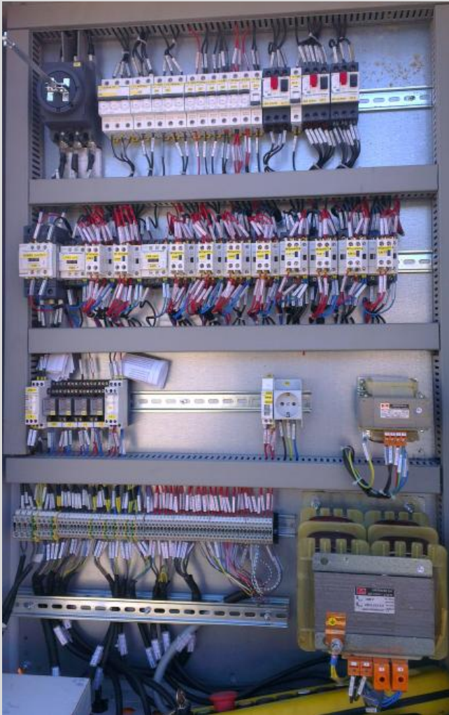
Electrical panels for crane with relay – contactors control and with frequency invertors in network communication with PLC.
